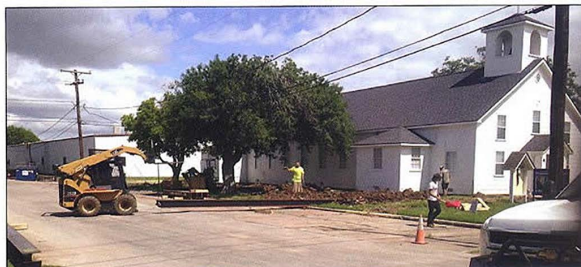
Cross loader beams being placed under structure.
