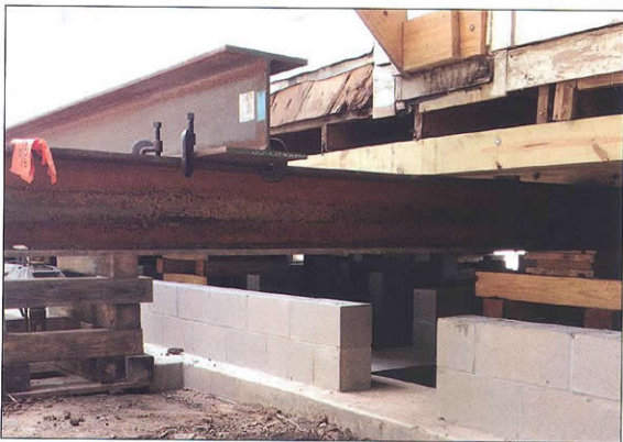
Notches in the new perimeter wall allows space for crossloaders to be removed when building is lowered.
