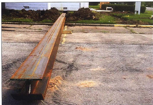
Cross loader beams being placed under structure.
