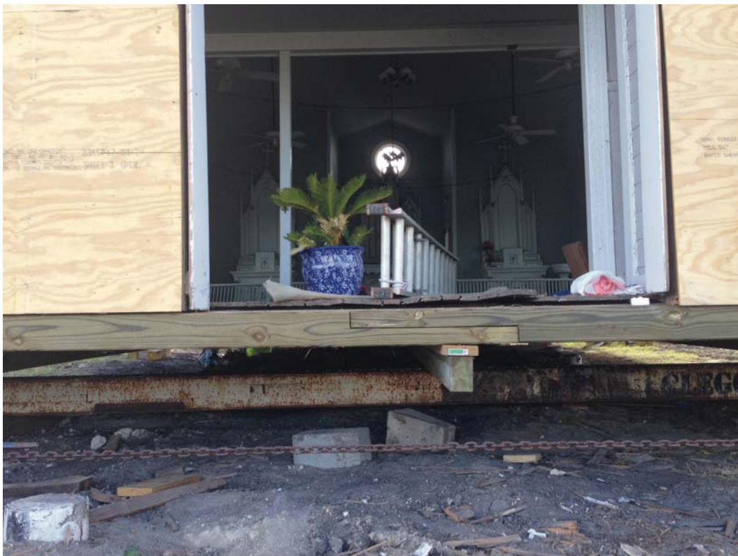
The Clegg Services crew lifted the church inch by inch with pump jacks and air bags until it was about 4 feet off the ground to do structural repairs underneath.
