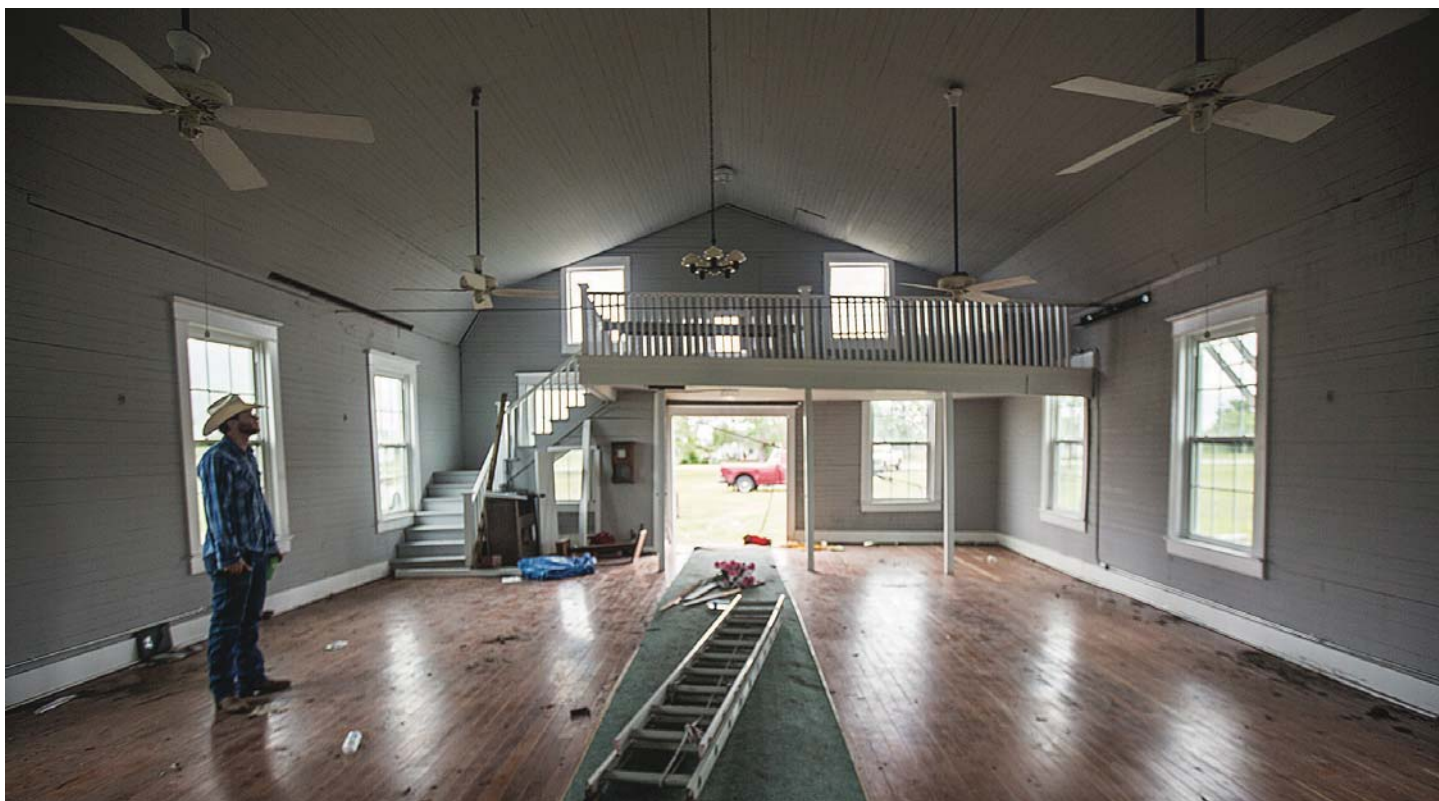
Mitchell Morrissey, 27, stands on the slumped floor of the Infant Jesus of Prague Catholic Church in McFaddin and looks at a cable wire strung through the walls. The cable is attached to a truck that helped level the church.
