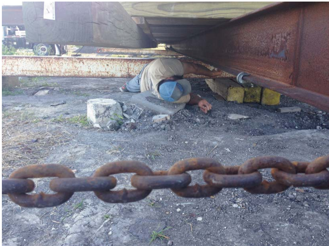
Gilbert Rodriguez with Clegg Services puts ivory soap on metal beams underneath the McFaddin church. Crews used the soap to help the church slide back onto its foundation.
