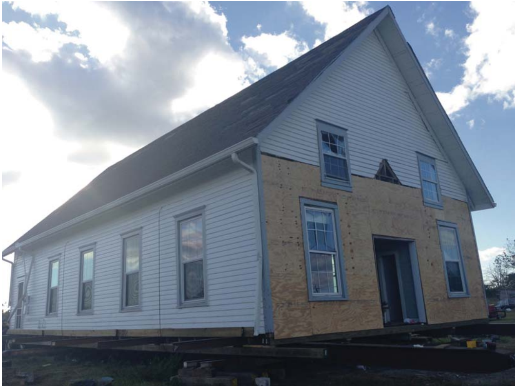
Clegg Services pulled the iconic McFaddin Church back onto its foundation. Hurricane Harvey blew the church about 15 feet of its foundation and caused the structure to lean at about a 30 degree angle.
