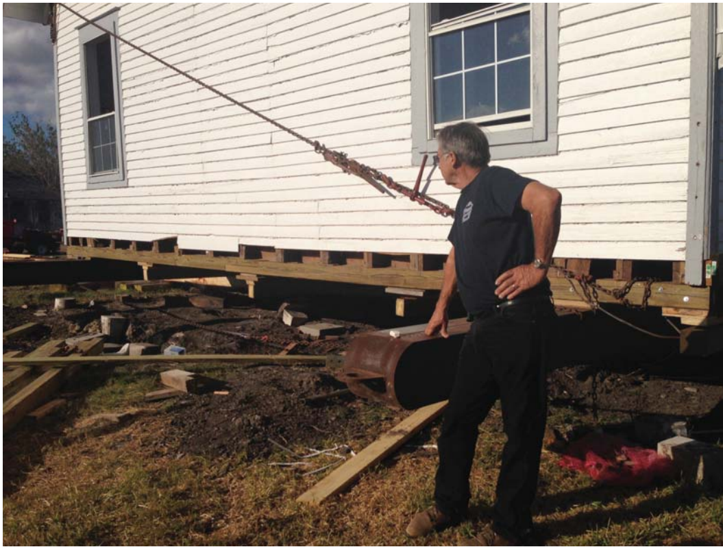
John Clegg, owner of Clegg Services, watches the McFaddin church move as its being pulled back onto its foundation.
