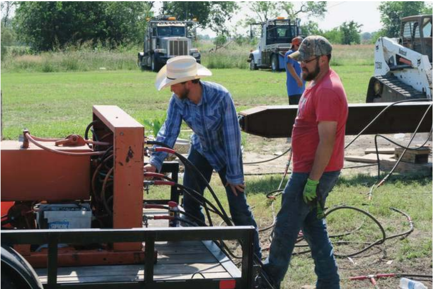
Mitchell Morrissey, of the McFaddin family, operates a pneumatic pressure lift to raise the Infant Jesus of Prague Catholic Church at the McFaddin ranch. Contributed by Gary Dunnam for The Victoria Advocate
